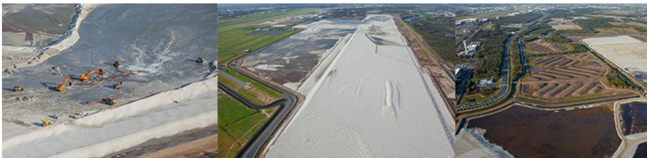
Figure: New parallel runway in construction
